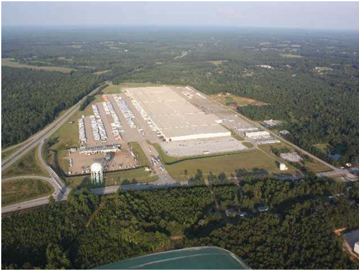
Wal-Mart Distribution Center
